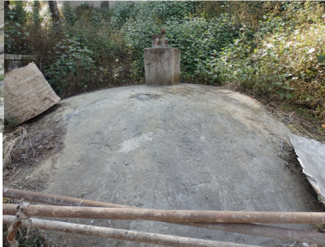
Dome of Biogas plant
