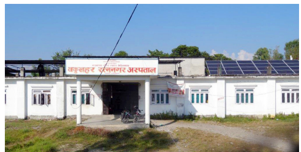
Solaranlage Ratnanagar Spital
